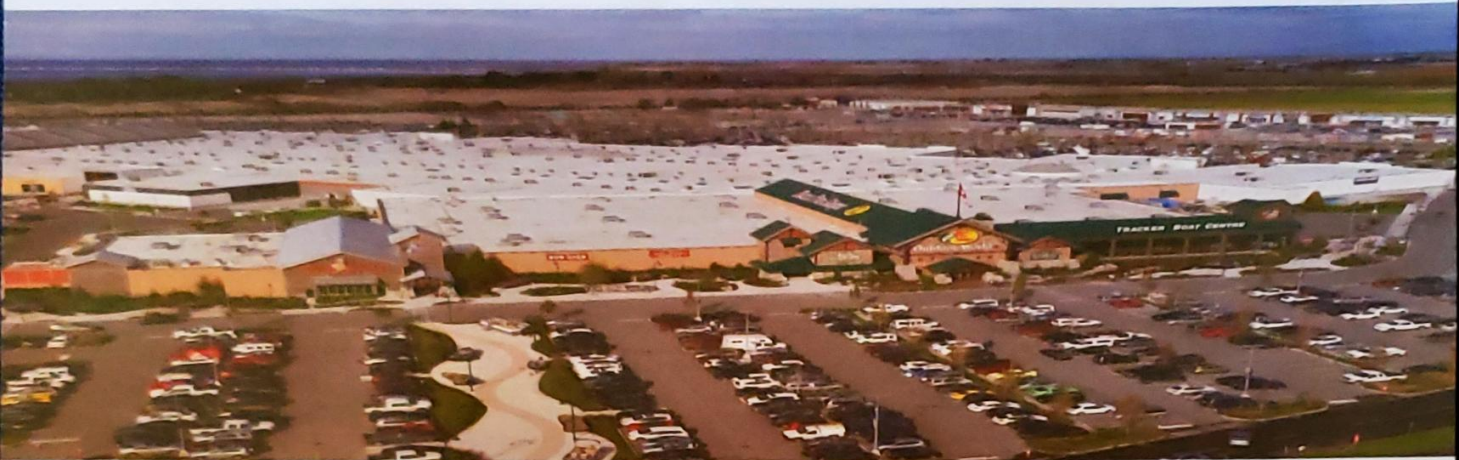
The $600-million Tsawwassen Mills shopping centre has 1.2 million square feet of retail space and a 1,100-seat food court
